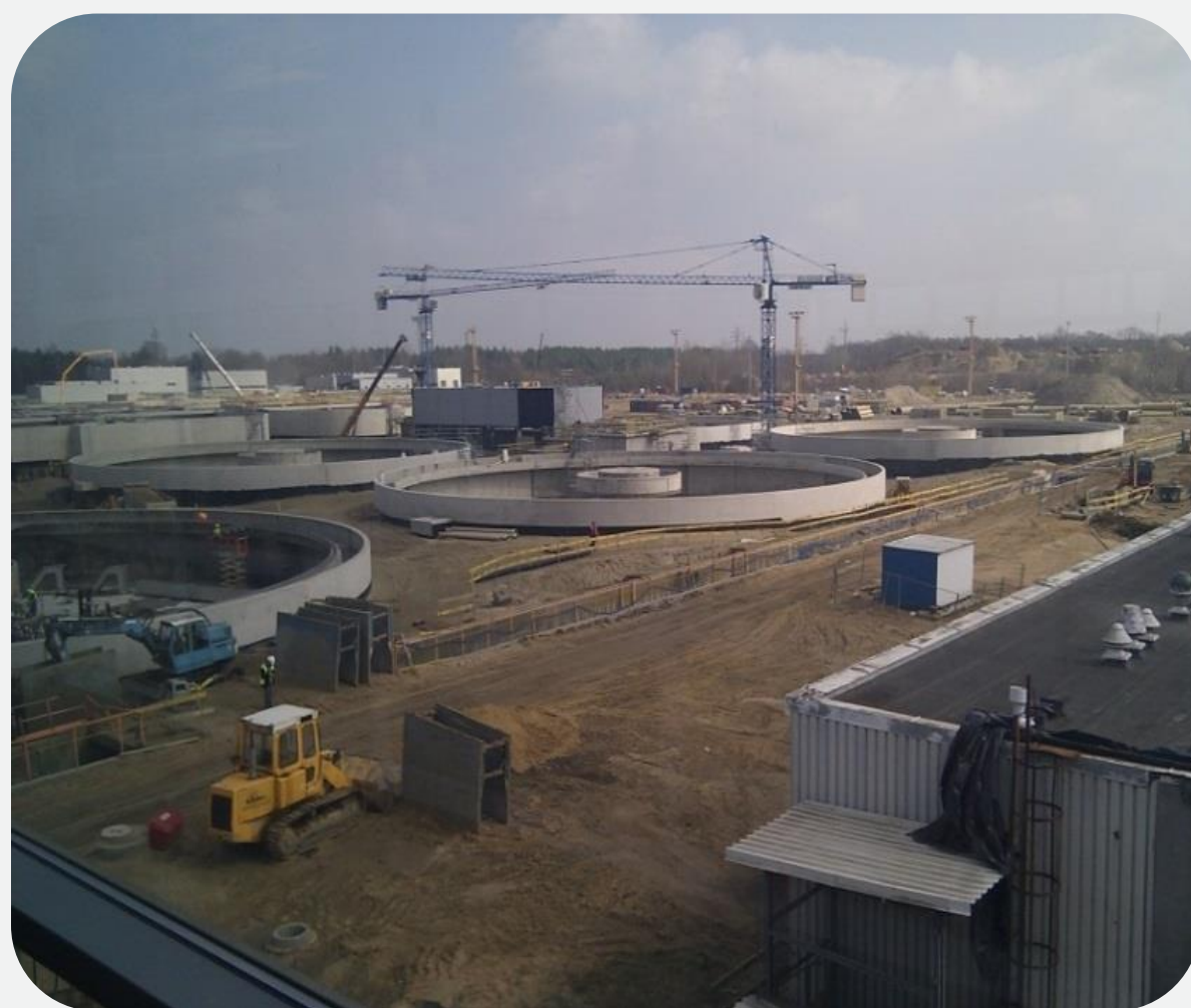
photo: waste water treatment plant Czajka, Warsaw, reconstruction 2009-2019
